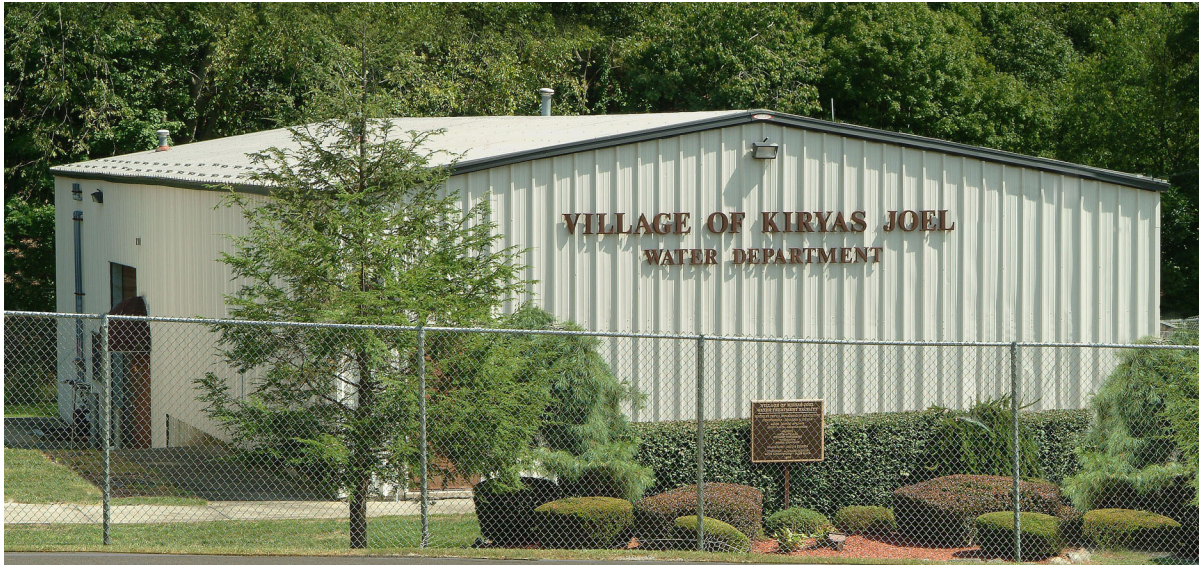
Kiryas Joel Water Plant
