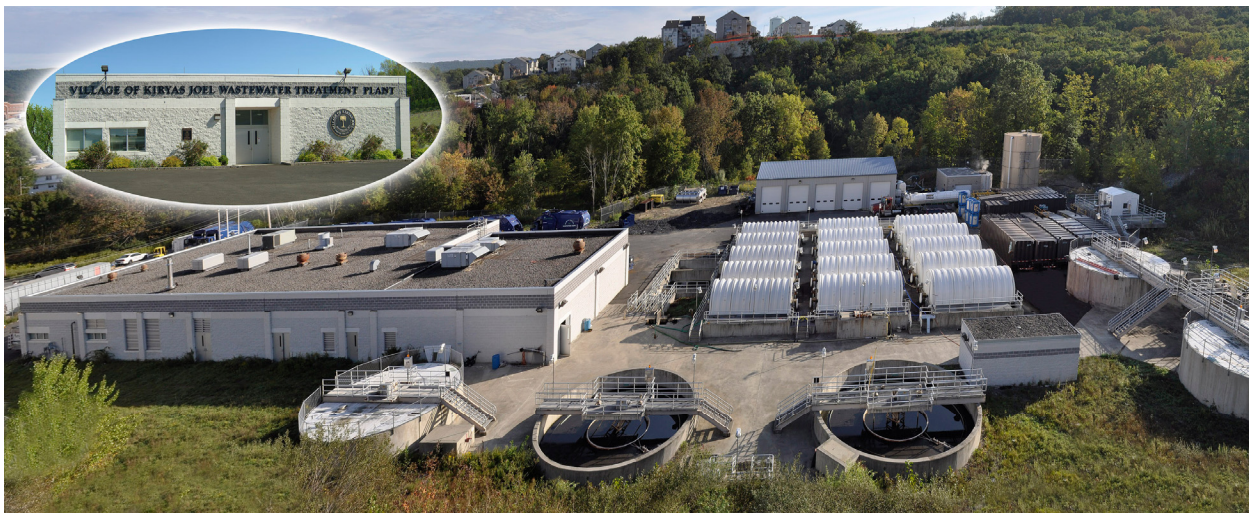
Kiryas Joel Wastewater Treatment Plant
